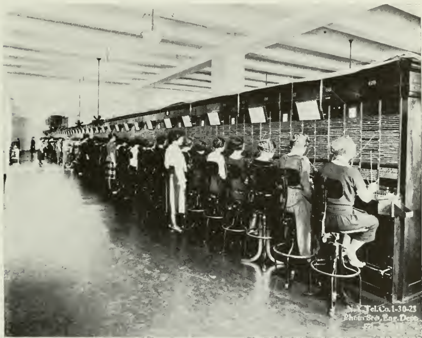
Fig. 2—Modern Type Common Battery Switchboard
