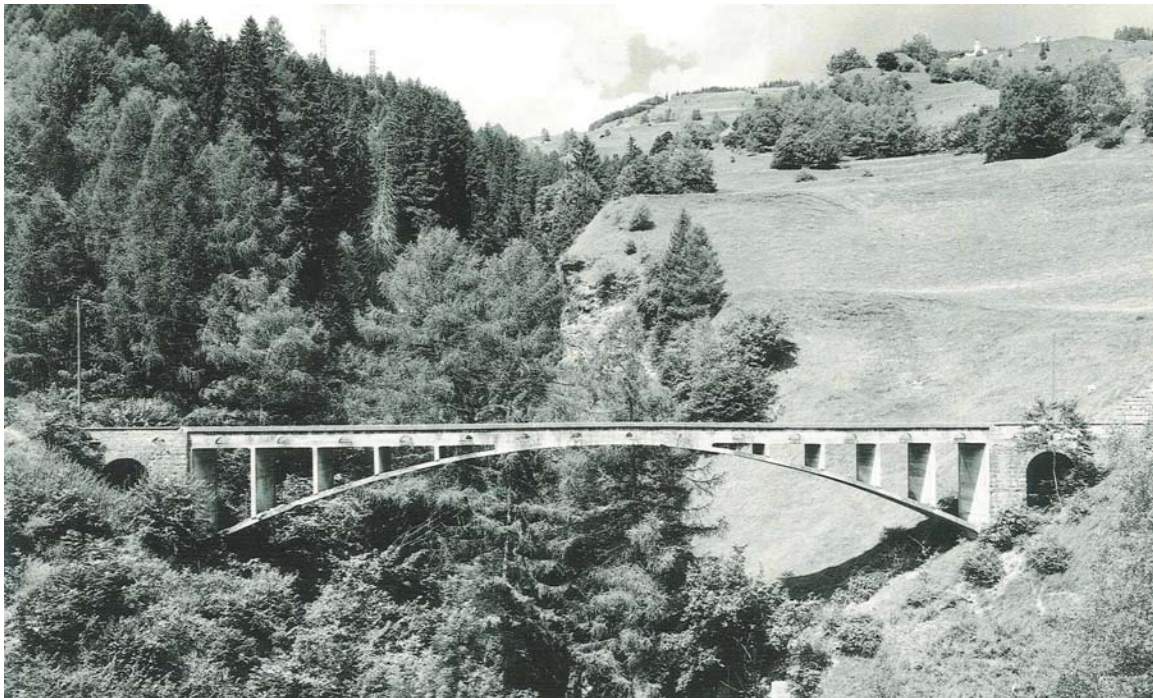
Figure 1. Robert Maillart's 1925 Valterschielbach Bridge in Switzerland (image credit: Billington 2005).
