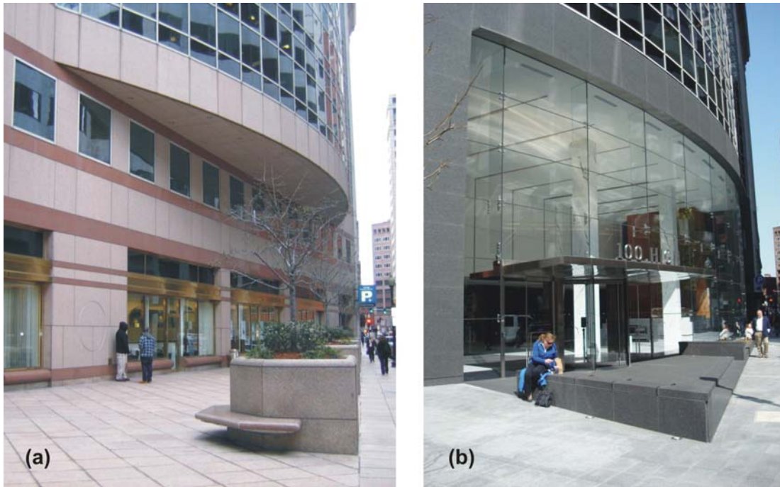
Figure 6. Lobby Renovation, 100 High Street, Boston, Massachusetts. (a) Before: two levels of retail space at base of 28 story building (photo credit: CBT Architects). (b) After: two-story lobby with structural glass wall hung from cantilevered third floor.
